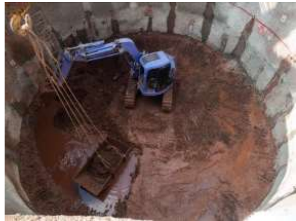
shaft excavation
