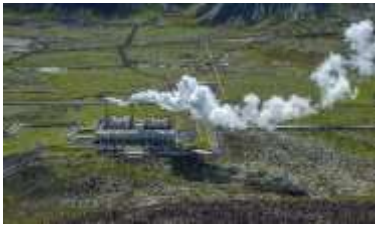
geothermal power plant-Iceland
